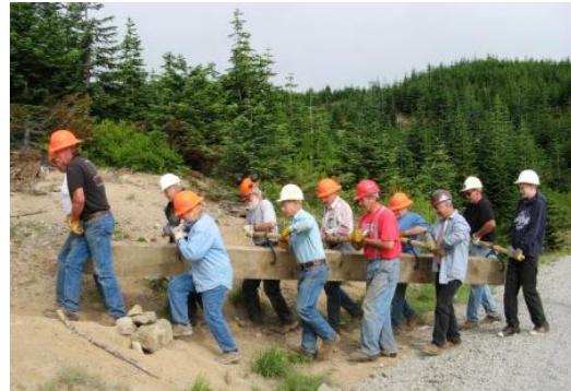
Placing a bridge stringer
